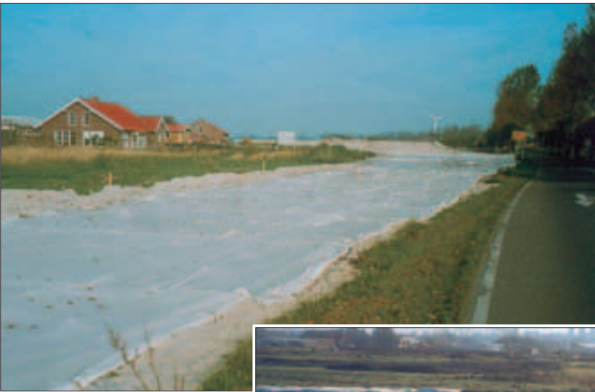
reinforcement with Stabilenka® 150/45 for the access to the Jever bypass, Germany
