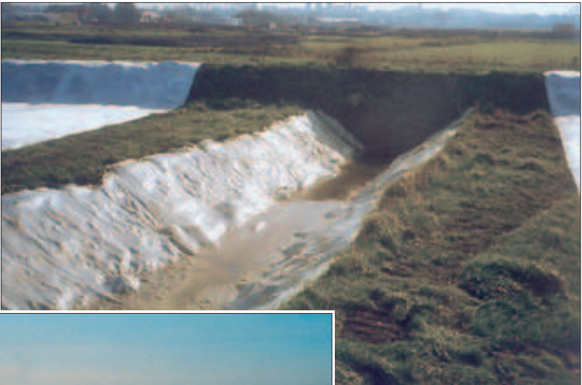
additional reinforcement to existing trenches
