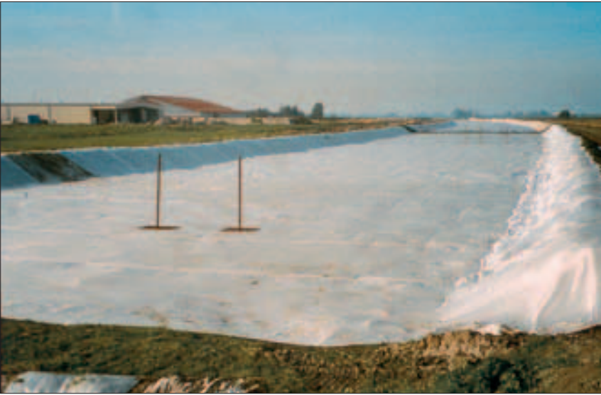
reinforcement with Stabilenka® 300/45 for the bypass embankment
