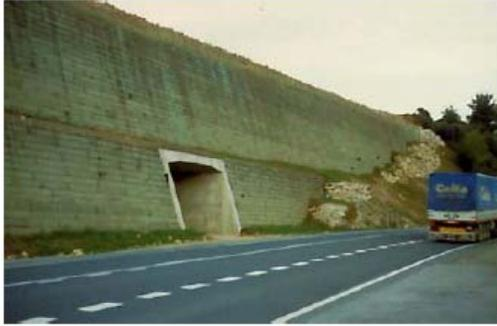
The finish of the outer face of the walls was more than satisfactory. The use of external shuttering of the Orleki type made this finish possible, at a very reasonable cost, and observing safety criteria for the operating staff.
