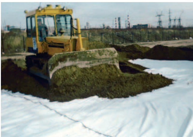
Placing the sand to form the capping
