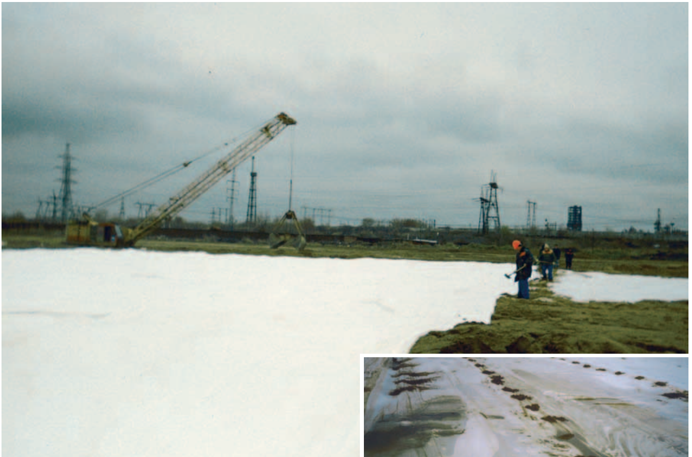
Laying the Stabilenka ® pieces
