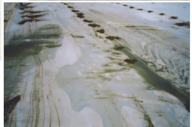
Stabilenka ® woven laid over the sewage sludge
