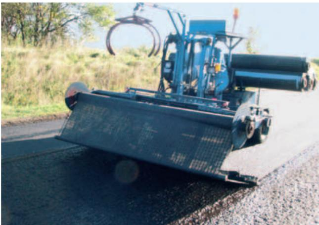
HaTelit® laid out immediately onto the sprayed, milled surface
