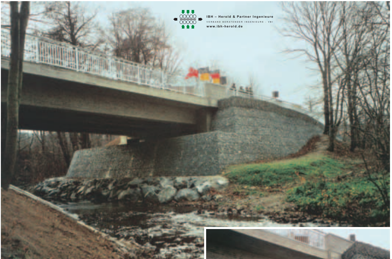
K 1355 bridge over River Ilse at Ilsenburg
